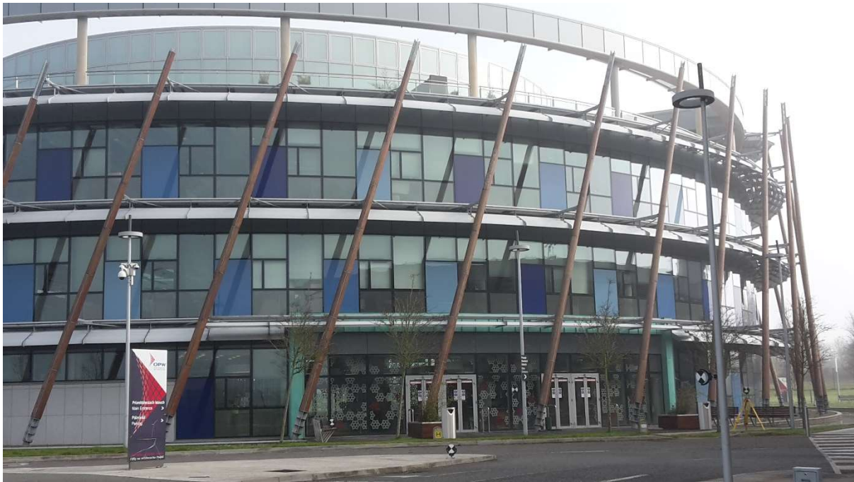
Facade of the OPW Head Quarter with black and white tilt-and-turn targets in front of it
